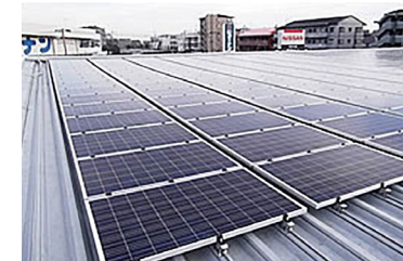
Solar panels on the roofs of some Kanagawa Nissan dealerships. Power from the panels is supplied to dealerships through the PPS system.
