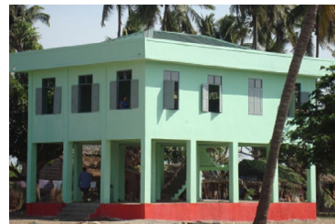
A school building can double as a disaster shelter in emergencies (construction planned in Myanmar).
